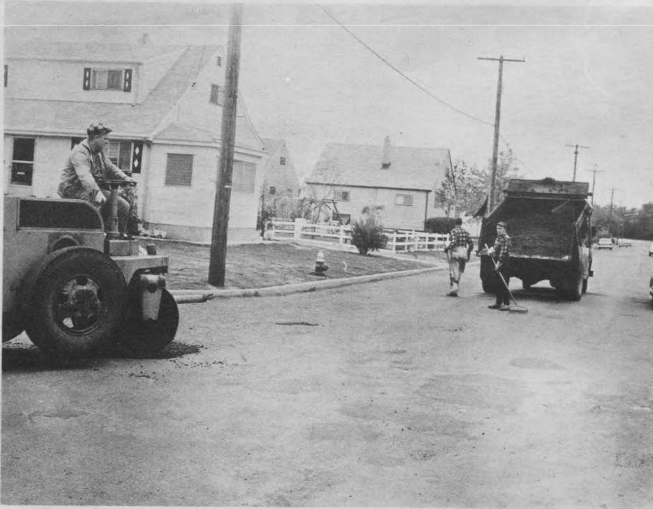
PATCHING UP: Township Road Department employees patch "pot holes". The roller presses the material into the holes. Ac-
